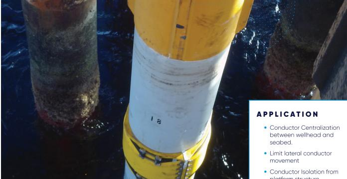
Conductors for fixed platform wells are typically installed through guidecans, which are part of the platform structure and placed at regular intervals between the well head and the seabed. Clearance of the conductor within the guide-can is required for installation but is not desired post installation. Matrix Composites & Engineering supplies Conductor Centralizers that are bonded to the conductor, centring the conductor within the guide-cans.
