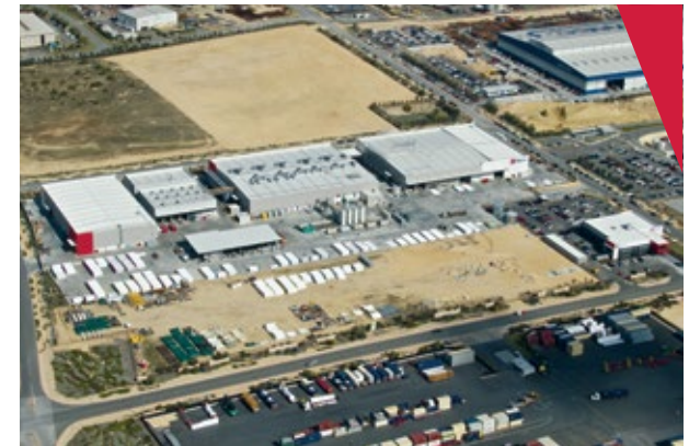
ABOVE: Matrix is located in the Australian Marine Complex, the southern hemisphere's premier integrated marine industrial facility
