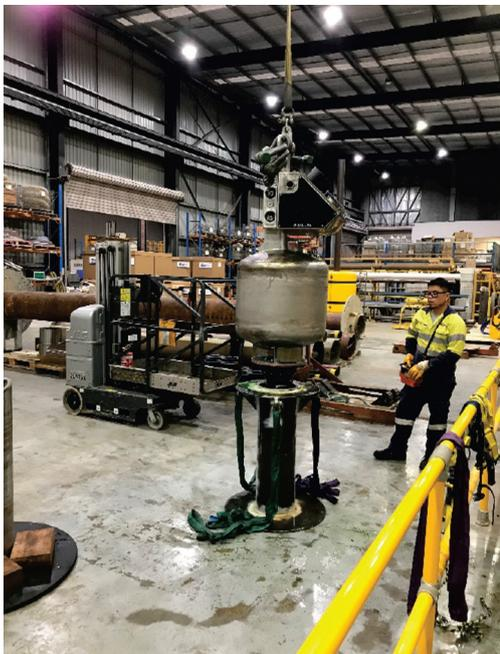
Subsea ROV Plug positioned and lowered into chamber.
