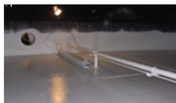
Interior crude oil storage tank
