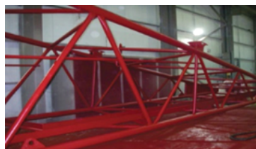
Offshore crane structure
